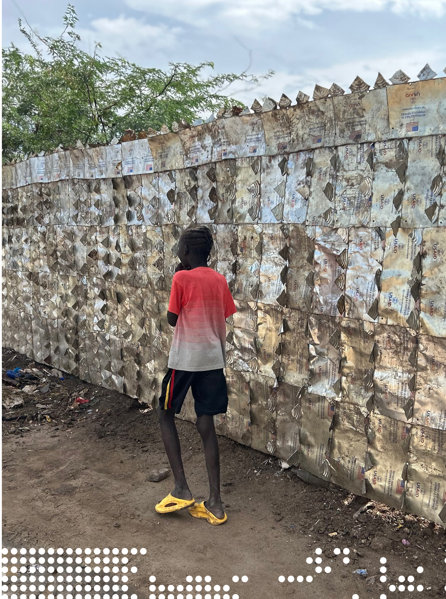
Fence in Kakuma Refugee Camp made of cooking oil containers provided on general food distributions @ Ayo Degett/DRC
