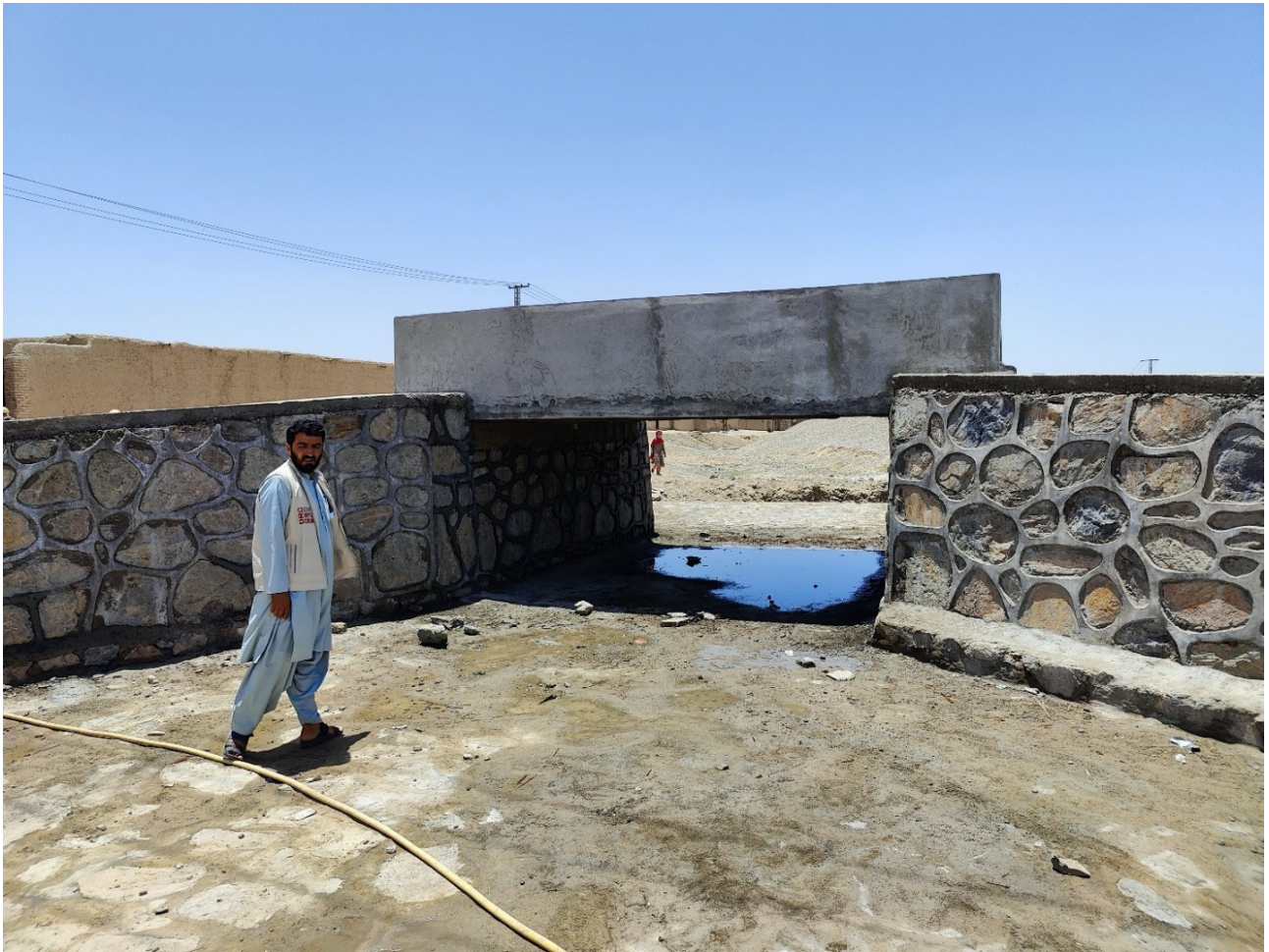
Culvert bridge build by DRC in an informal settlement in Kandahar
